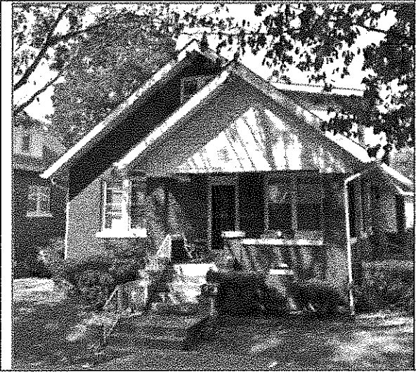
917 12 th Street (Front View)
