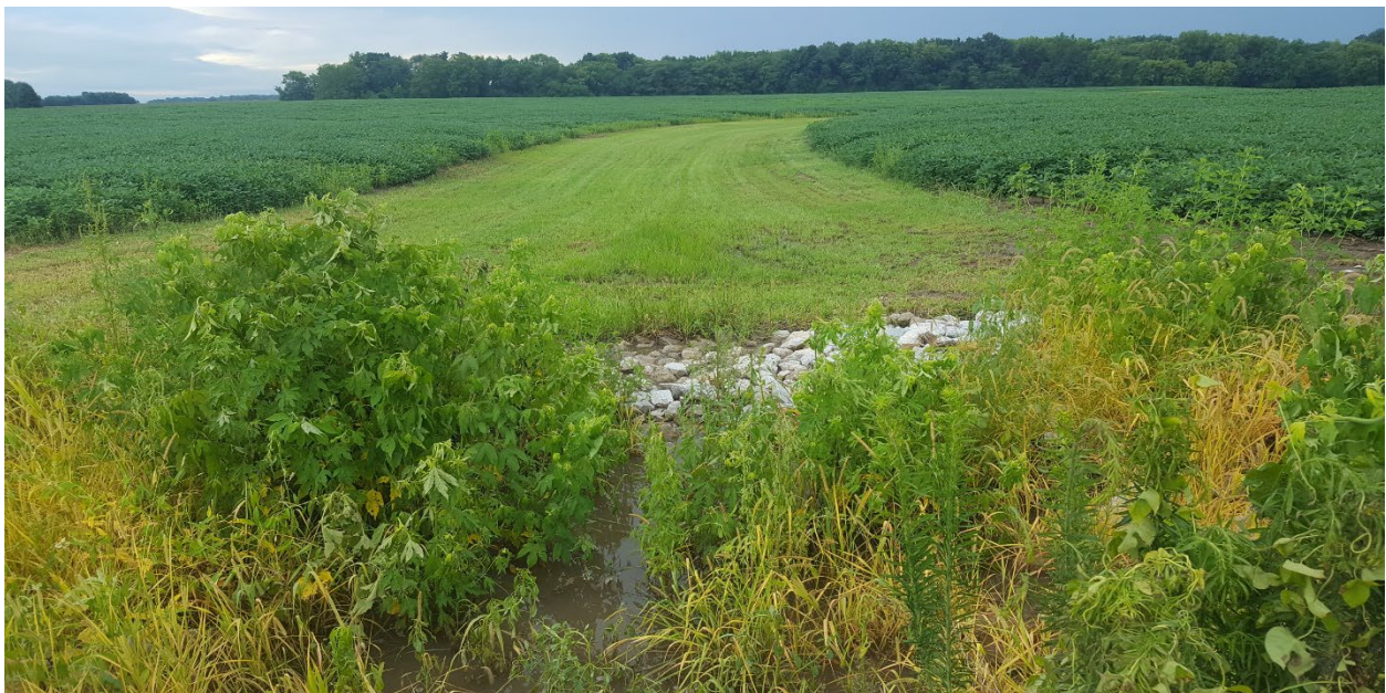
Grassed waterway installed in Highland Silver Lake watershed
