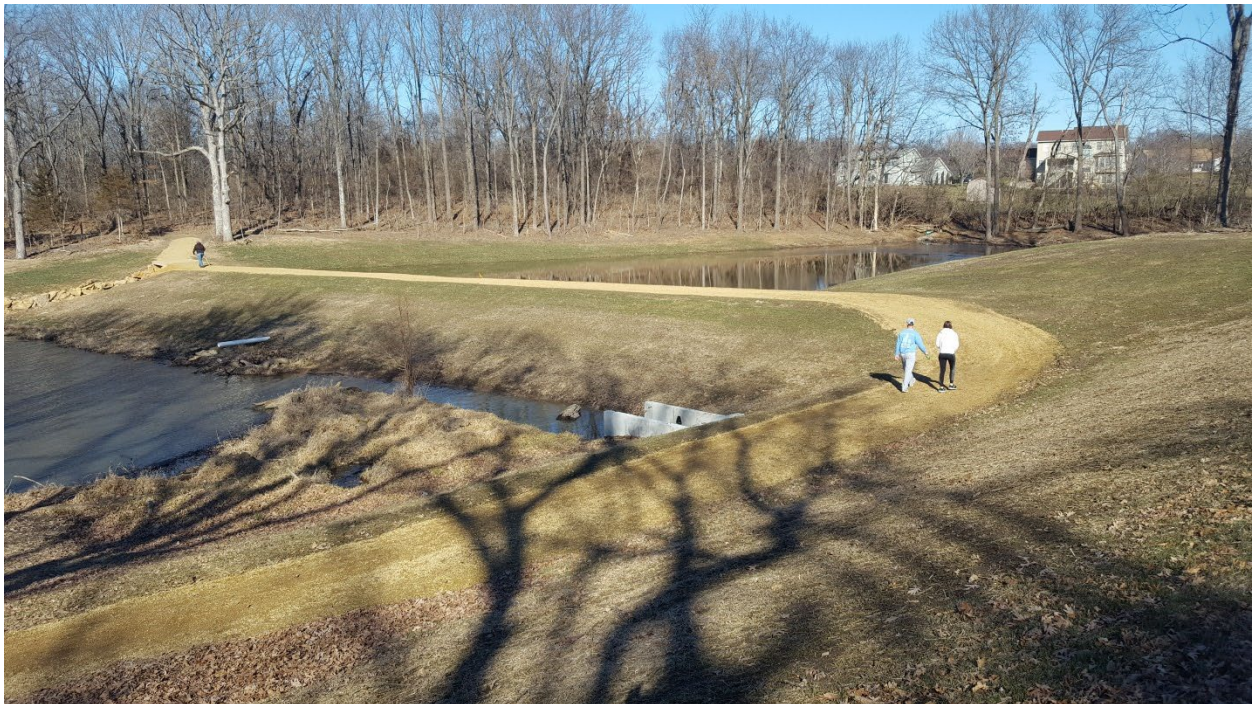
Image: Constructed wetland in Highland Silver Lake Park
