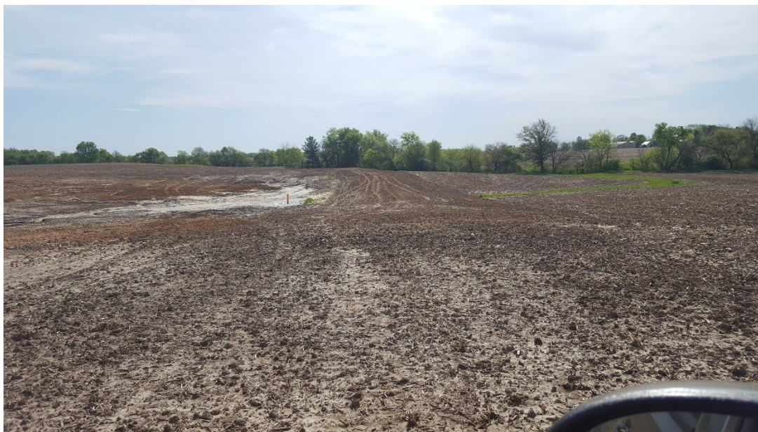
Water and sediment control basin installed in Highland Silver Lake watershed
