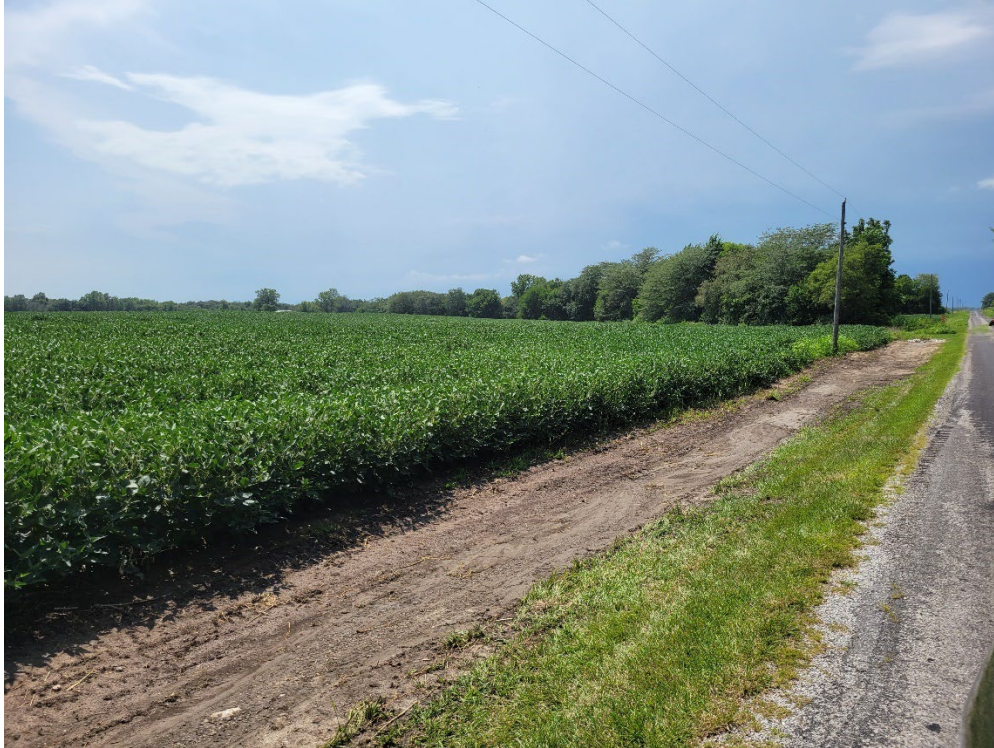
Reshaped roadside drainage ditch installed in Highland Silver Lake watershed
